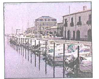
From £251,000: 12 apartments on the waterfront in Marseillan, Languedoc. Through Garrigae (00 33 467 118757)
